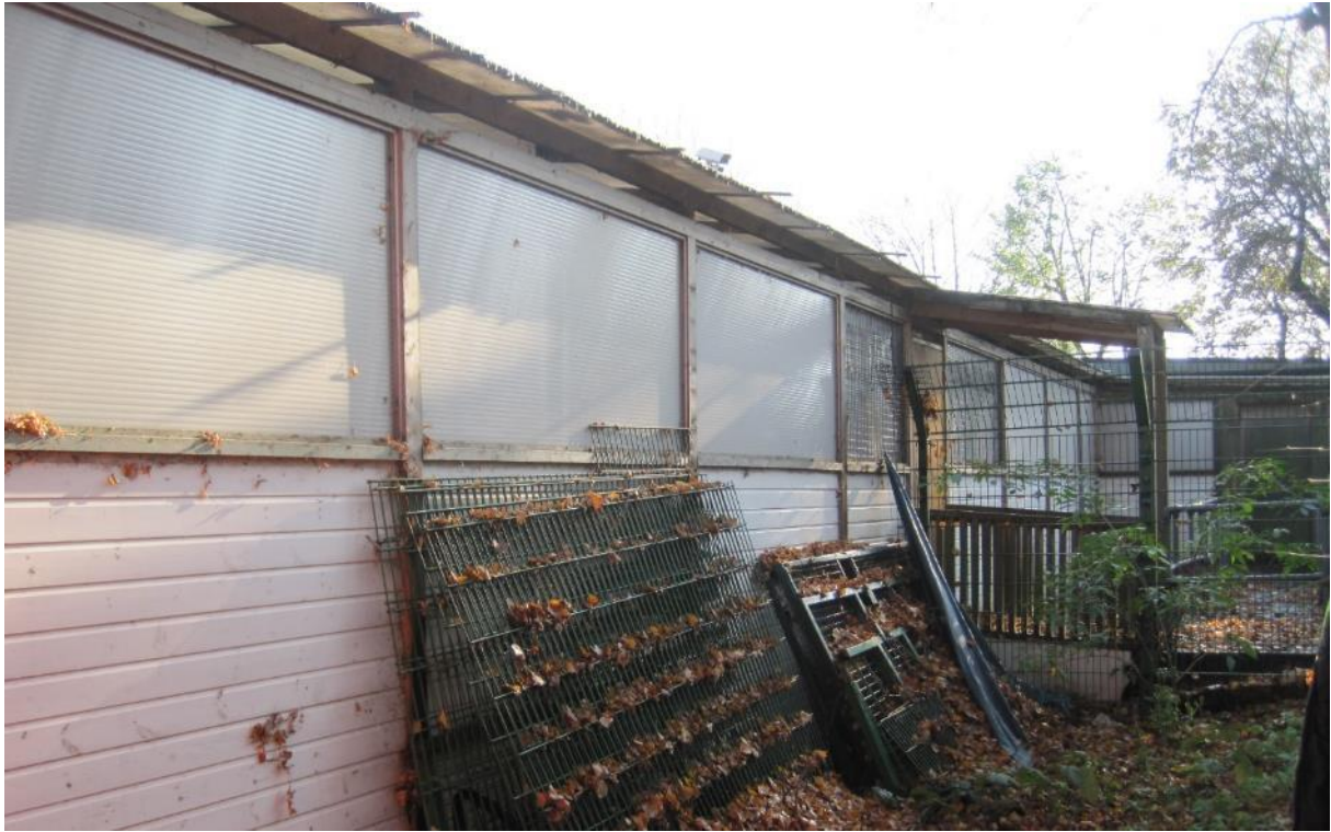
Figure 6.2: The temporary building added to the west end of the school
