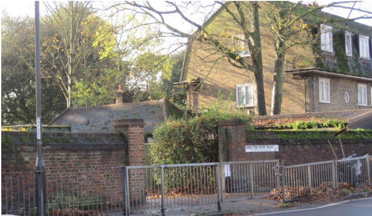
Figure 5.5 Start of the listed wall on Charlton Park Road opposite Charlton Lane, east of this point the wall continues in part as the boundary to Mulberry Close the 1960s flats seen on the right.
