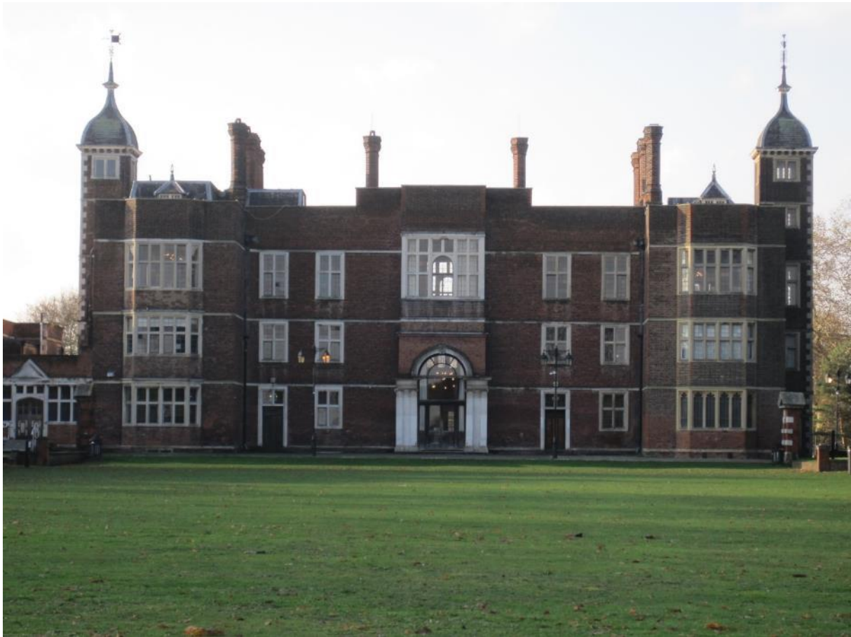
Figure 5.2: East elevation viewed from the ha-ha with the link range to the stables at the south end
