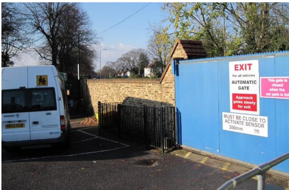
Figure 5.7 The listed wall within the school showing its setting. The van is where the new building will be
