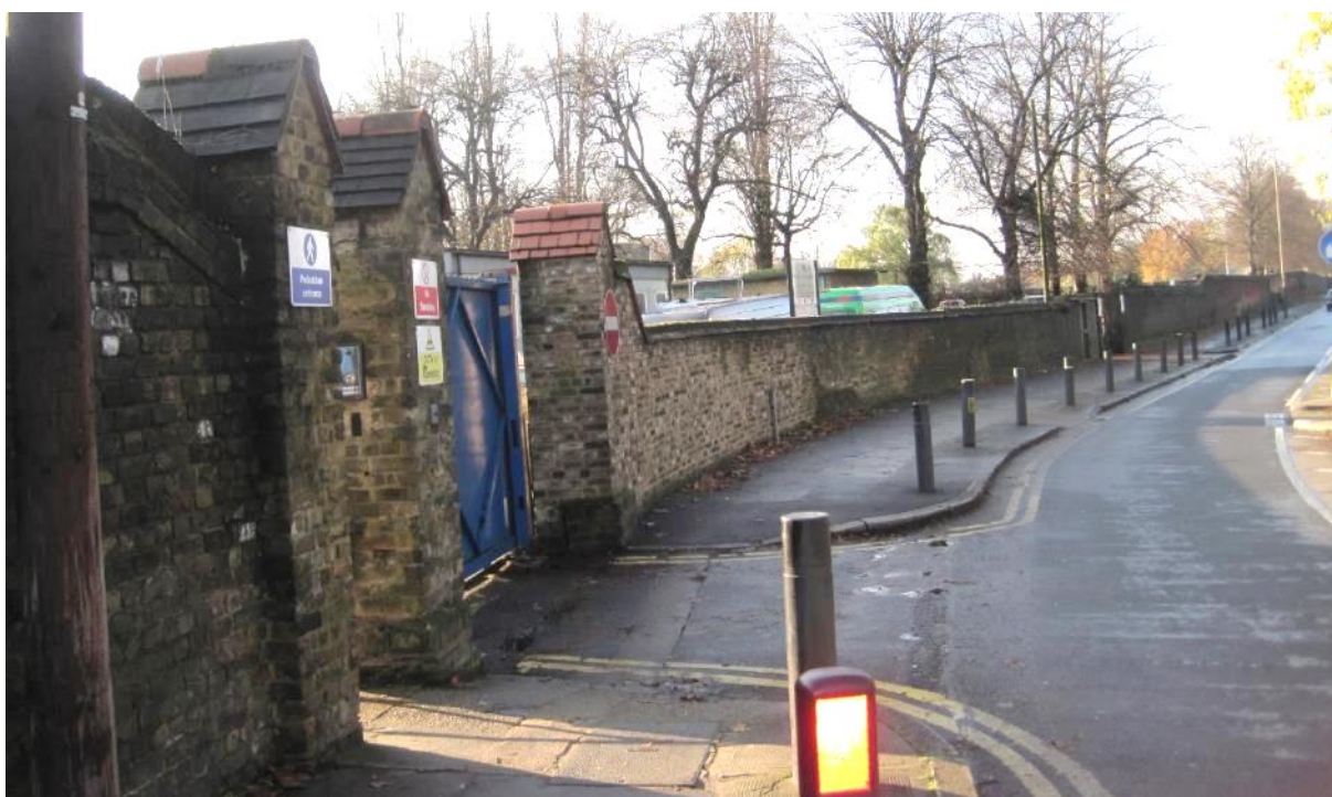
Figure 5.4: Wall at the Site (only partially visible).
