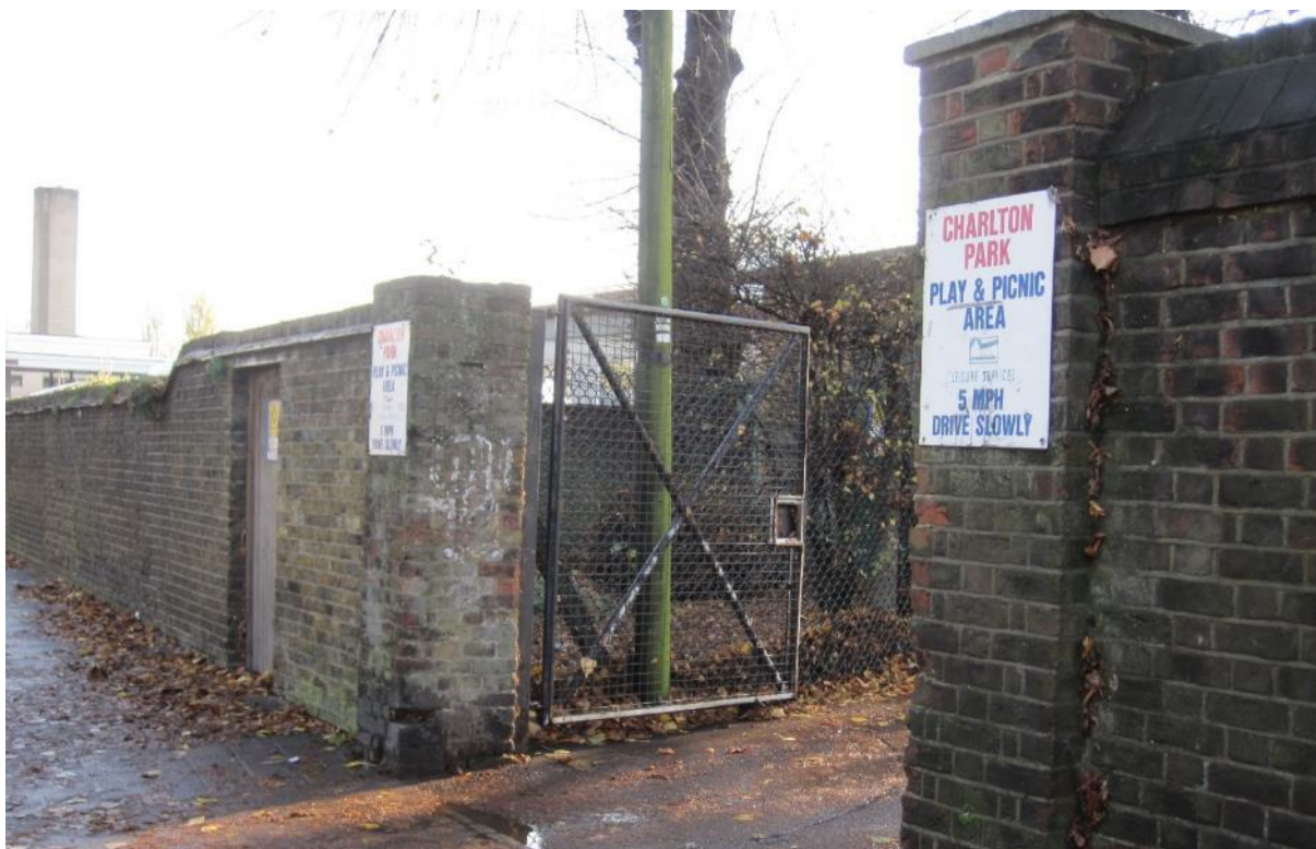
Figure 5.3: Wall at entrance to sports pavilion and horse manège, with the electricity sub-station and then site behind it on the left. The raised section of wall demarcates the sub-station enclosure.
